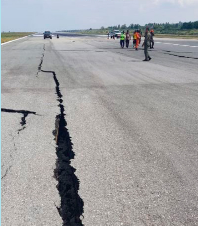
▶ Photos top to bottom, left to right: Indonesian air traffic controller Anthonius Gunawan Agung, Indonesian military personnel carry Agung's remains during his funeral, the cracks from the earthquake in a runway at Mutiara SIS Al-Jufrie Airport near the city of Palu, the collapsed air traffic control tower at the airport.
